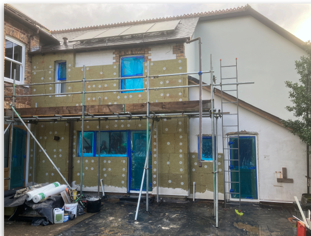
Figure 3 Insulation slabs being fixed
