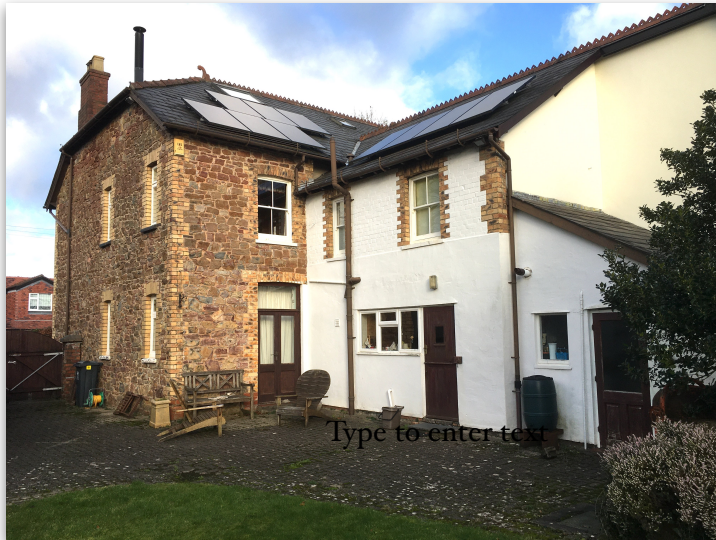
Figure 1. The rear of the house in January 2022 before the window replacement
