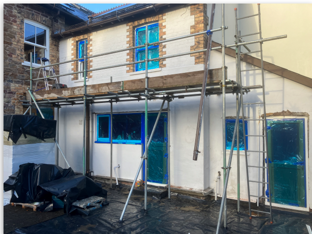
Figure 2 Scaffolding in place and the paving, windows and doors protected
